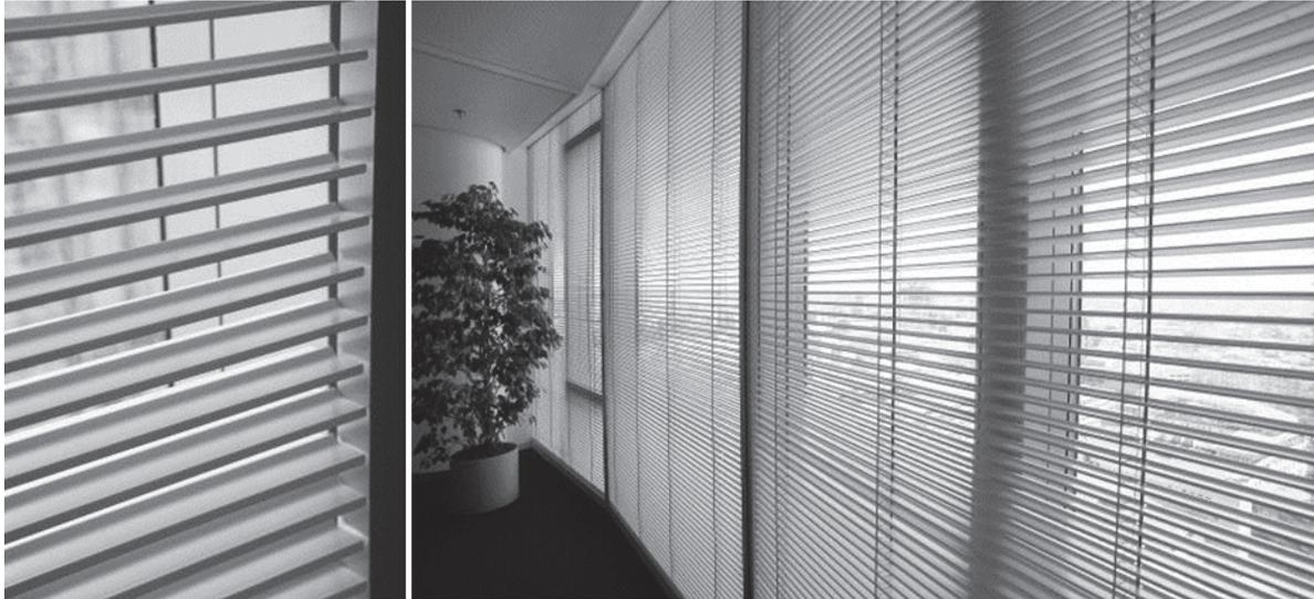
Figure 61: Internal venetian blind with 'Genius slats' in the 56-storey building Main-Tower in Frankfurt(Main), Germany. The original internal venetian blinds with mirror finished surface have been replaced since 2008 step by step by venetian blinds with genius slats in order to avoid overheating [124].
