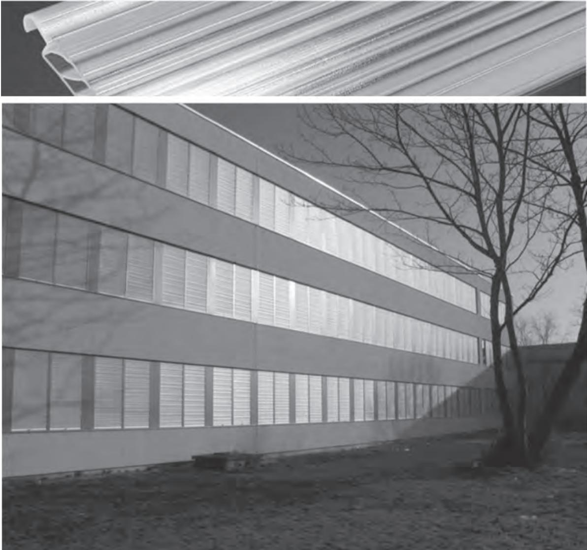
Figure 63: Daylighting roller shutter, viewed from outdoors. A cross-section of the translucent lath can be seen in the upper illustration. The new laths were developed by the author. Photos ©Prokuwa Kunststoff GmbH, Dortmund
