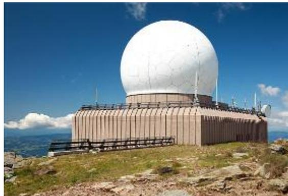
**Image 14: Radome on a ground station**
