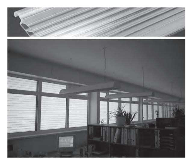
Figure 64: Daylighting roller shutter, seen from indoors. On the top, a cross-section of the translucent lath can be seen. Photos ©Prokuwa Kunststoff GmbH, Dortmund
