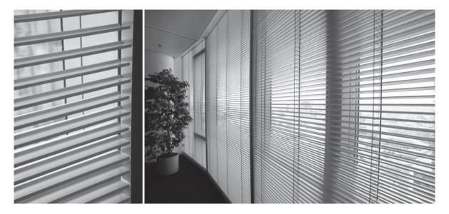
Figure 61: Internal venetian blind with 'Genius slats' in the 56-storey building Main-Tower in Frankfurt(Main), Germany. The original internal venetian blinds with mirror finished surface have been replaced since 2008 step by step by venetian blinds with genius slats in order to avoid overheating [124].
