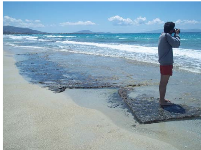
Figure 52: Signs of quarrying (rectangular cuts) in the shallower beachrock slab, in Mikri Vigla (W Naxos).
