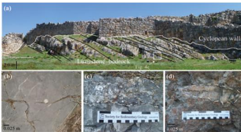
Figure 3.5.2: (a) Photo of western flank of Tiryns (looking east) showing the fortification walls erected on bedrock (white solid line marks the contact), subvertical joints (white dashed lines) and bedding (black solid lines). (b) Typical sedimentary structures in the bedrock include fine-grained calcite veinlets, (c) coarse-grained calcite veins, (d) geopetal structures, according to (Hinojosa-Prieto et al. 2015).
