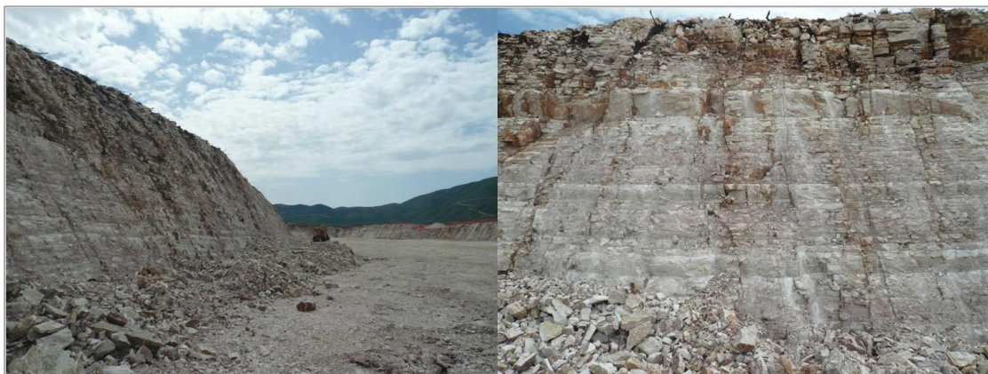
Figure 8. The road section from which samples were collected to be studied.
