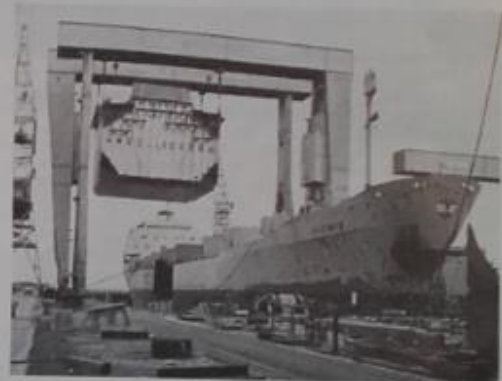
Left. The new 550-ton 20 m. section being lifted into place in one piece
