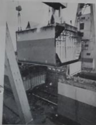
Left. The new 550-ton 20 m. section being lifted into place in one piece
