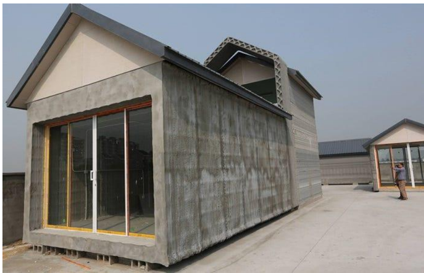
Fig. 29 3-D printed house by Winsun Decoration Design Engineering Co. with the help of contour crafting. [Levy Karyne et al., 2014]
