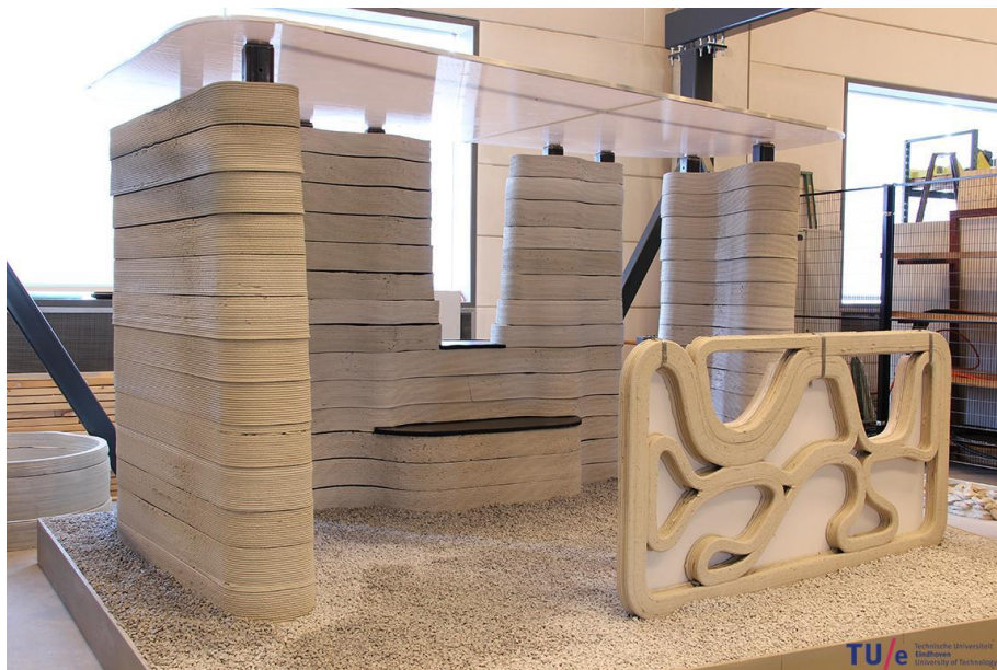
Fig. 36 Pavilion constructed by Concrete Printing. [Bridget B M. et al., 2016]
