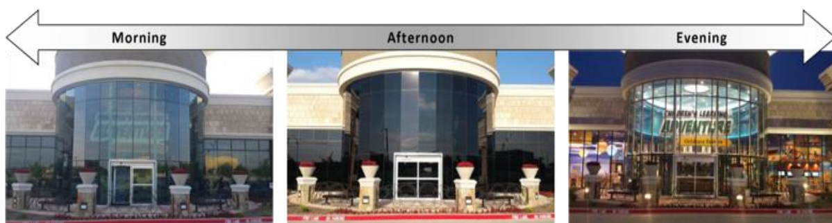
Fig. 6 Thermochromic glass windows installed at an educational facility in Keller, Texas, USA. [Source: Pleotint, LLC]
