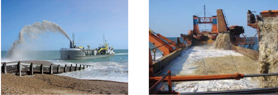
Figure 1.6. a) Marine aggregates pumped from the ship onto the beach (Eastern Solent Coastal Partnership, www.escp.org.uk ) and b) marine aggregates dredging on board (Marine Aggregates Dredging, www.hrwallingford.com ).
