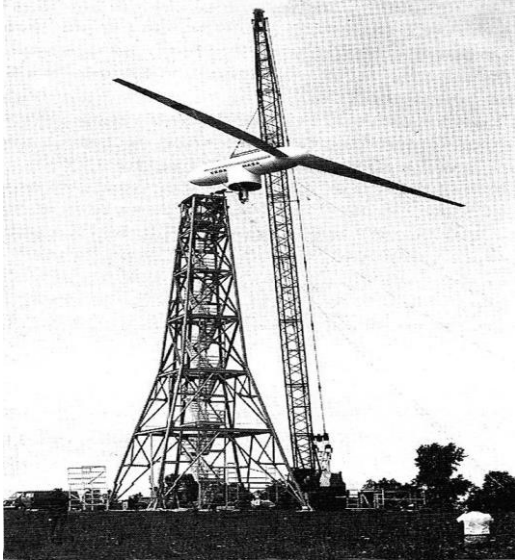
Figure 18: Final assembly of the 100 kW Mod-0 HAWT test bed in 1975. It was located at the NASA Lewis Plum Brook Test Station near Sandusky, Ohio. 41
