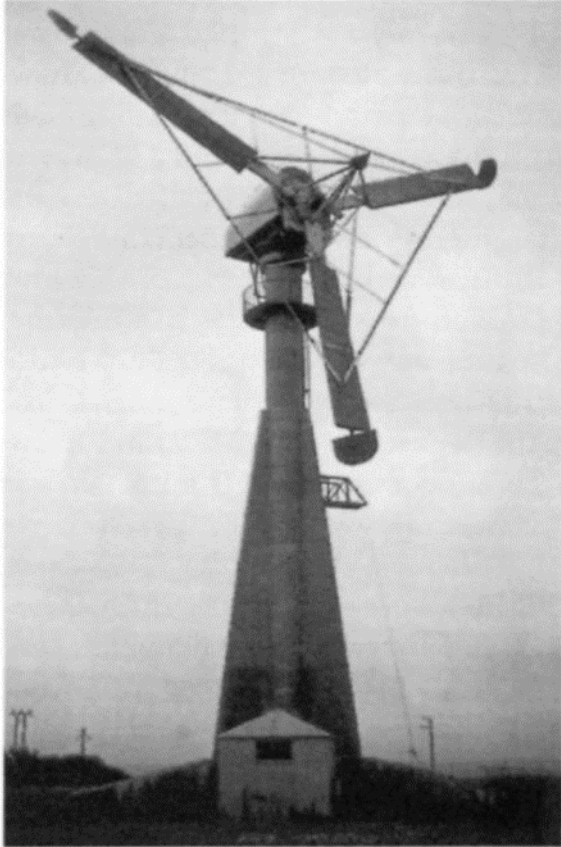
Figure 11: Johannes Juul's Gedser turbine with 200-kilowatt capacity, 24-meter diameter rotor and 25-meter tower height. 34
