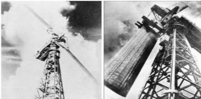
Figure 10: Smith-Putman's 1.25 MW wind turbine. Smith-Putnam wind turbine, the world's first MW-size wind turbine in 1941, installed in Grandpa's Knob in Castleton, Vermont, USA (Photos: NREL/DOE). 32
