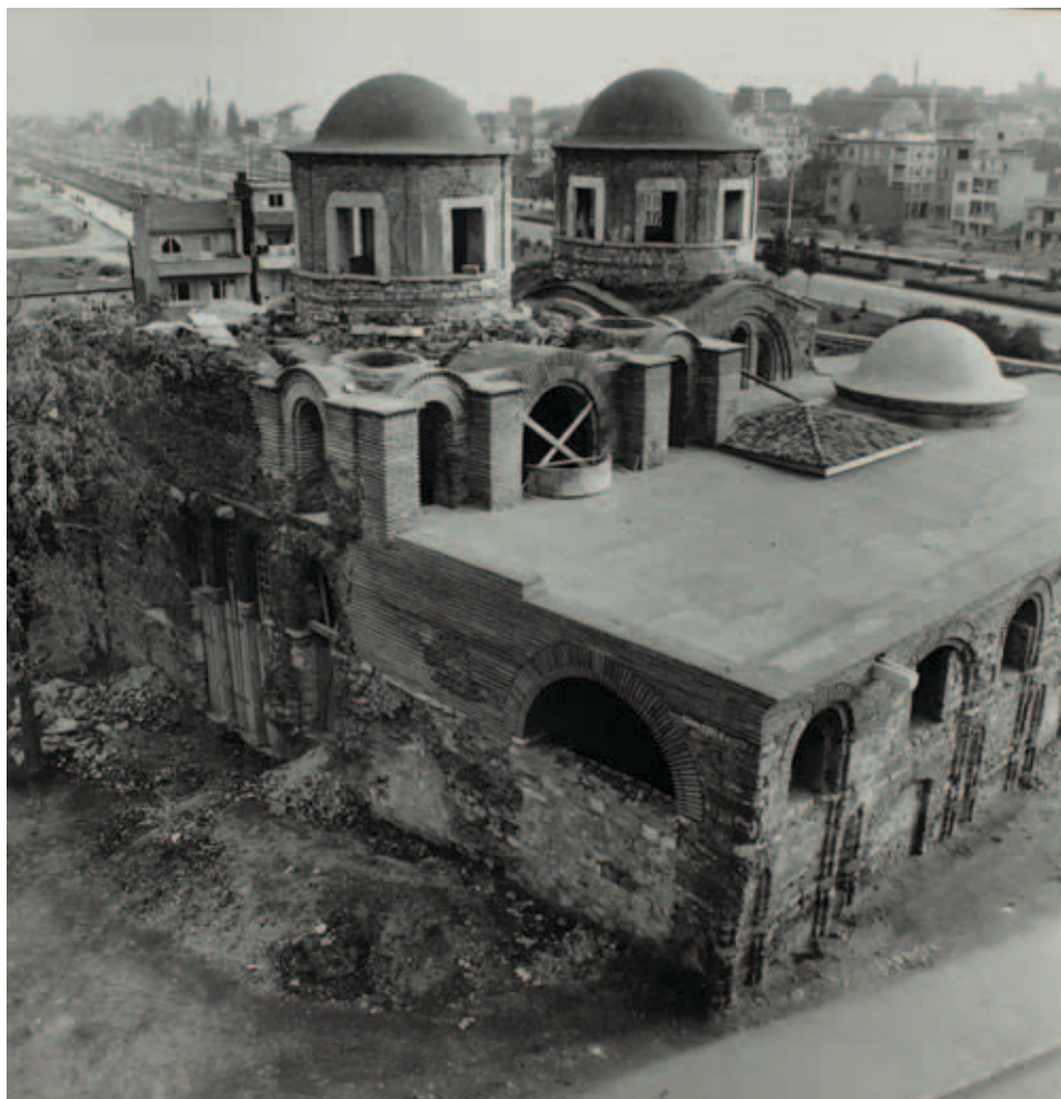
Fig. 10: Monastery tou Libos, view of the complex from the northwest after restoration, ca. 1963. © Dumbarton Oaks, Image Collections and Fieldwork Archives, Washington, D.C.
