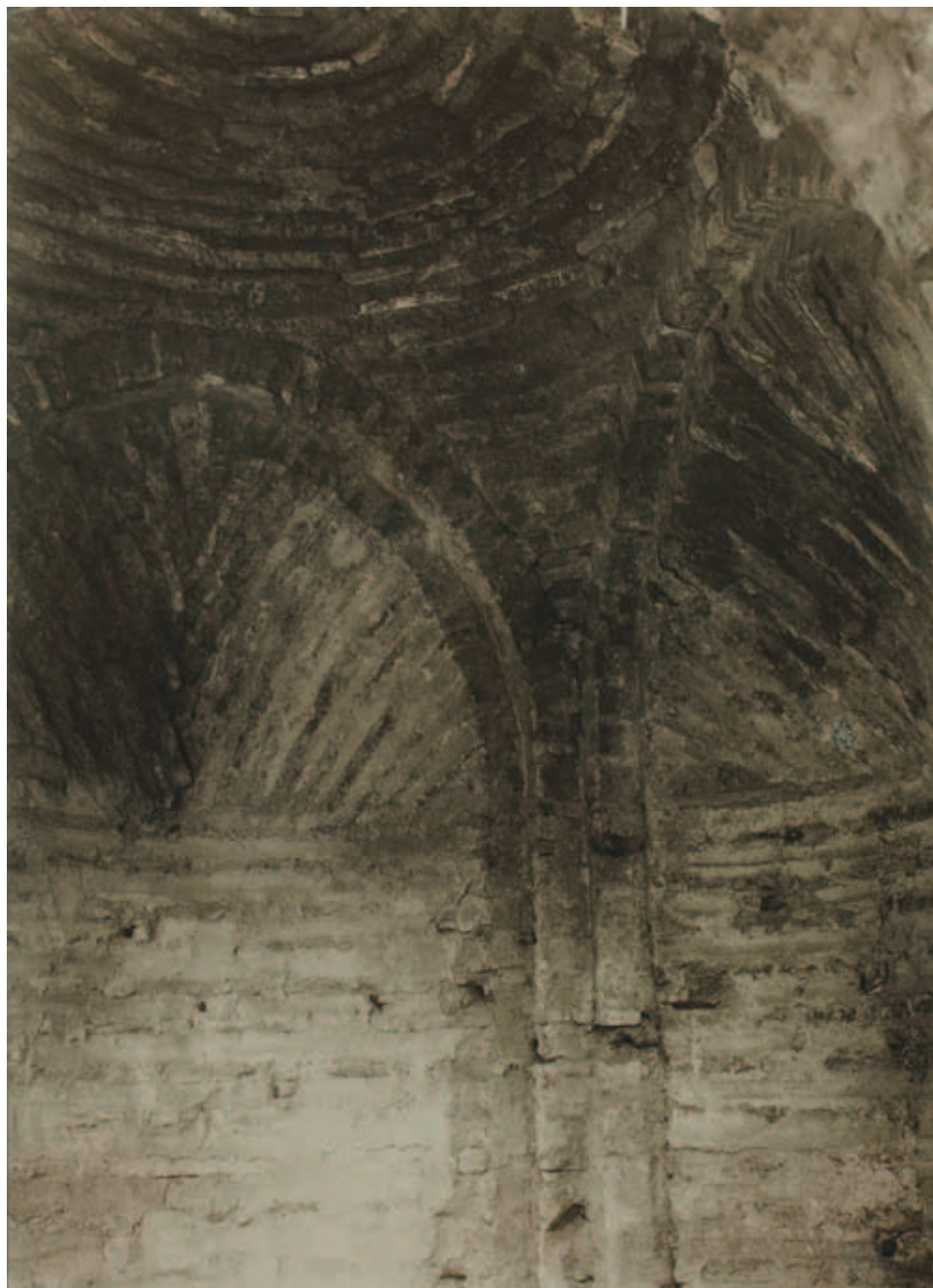
Fig. 18: Theotokos tou Libos, interior of the antechamber of the southeast roof chapel showing the domical vault. © Dumbarton Oaks, Image Collections and Fieldwork Archives, Washington, D.C.
