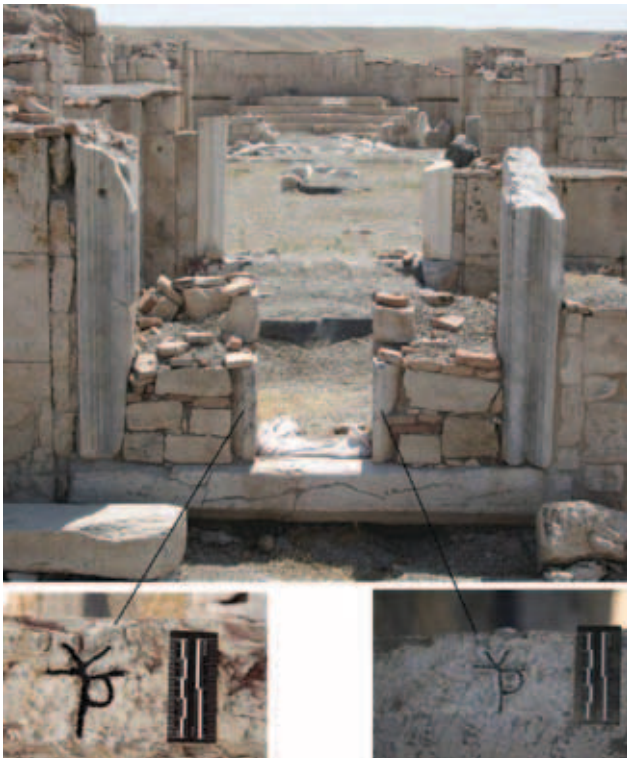
Fig. 7a-c. Amorium. West entrance of Basilica A, showing two Ionic impost capitals (T2454 and T2455) in secondary use and details of the masons' mark on their impost stones. Photos © Amorium Excavations Project.
