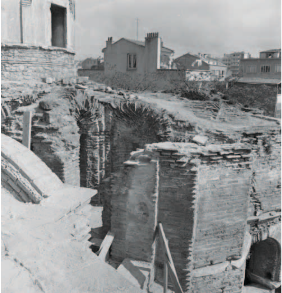
Fig. 15: Theotokos tou Libos, southeast roof chapel, ca. 1960. © Dumbarton Oaks, Image Collections and Fieldwork Archives, Washington, D.C.
