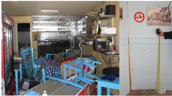
Figure 8.11. Site V2. Indoor material damage caused by the tsunami attack in the fish restaurant (a). Water mark at h \sim 1.09 m was measured at run-in distance of \sim 45 m (b) (photos credit, I. Triantafyllou).
