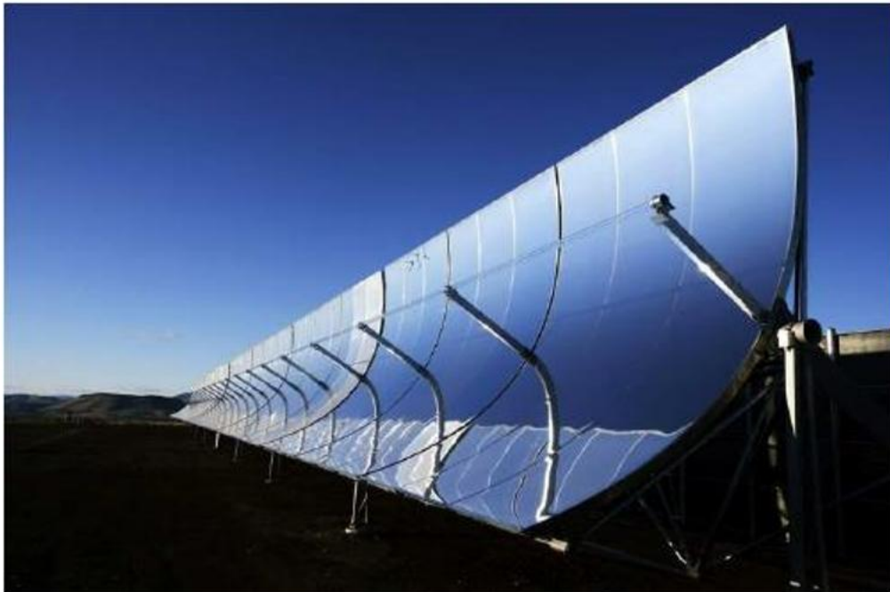
Εικόνα 124: Parabolic Trough - Concentrated Solar Power (Oil-Gas Portal – Solar Power Concentration)
