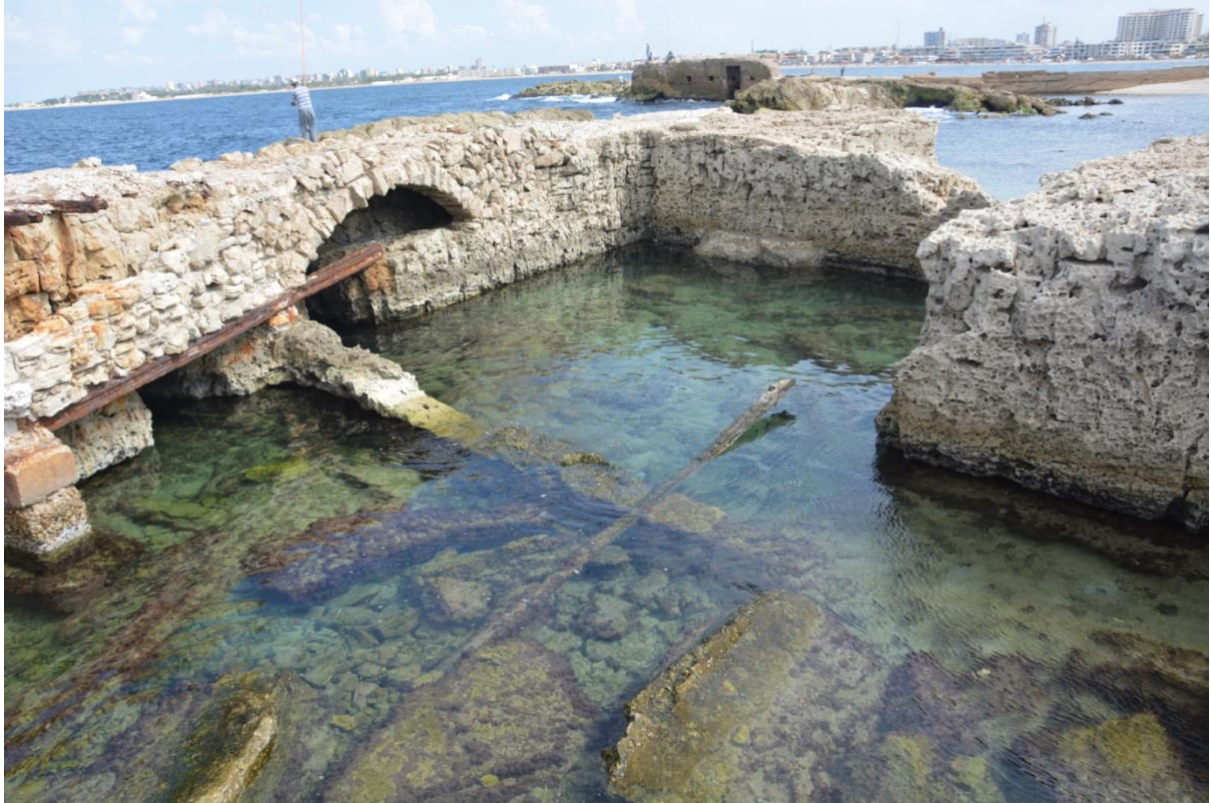
Montaza fish tank (view of the interior space)
