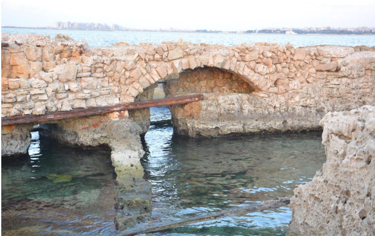
Internal of Montaza fish tank
