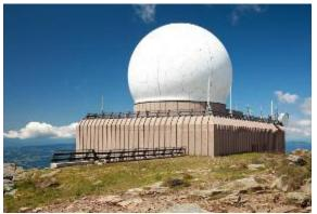
Image 14: Radome on a ground station
