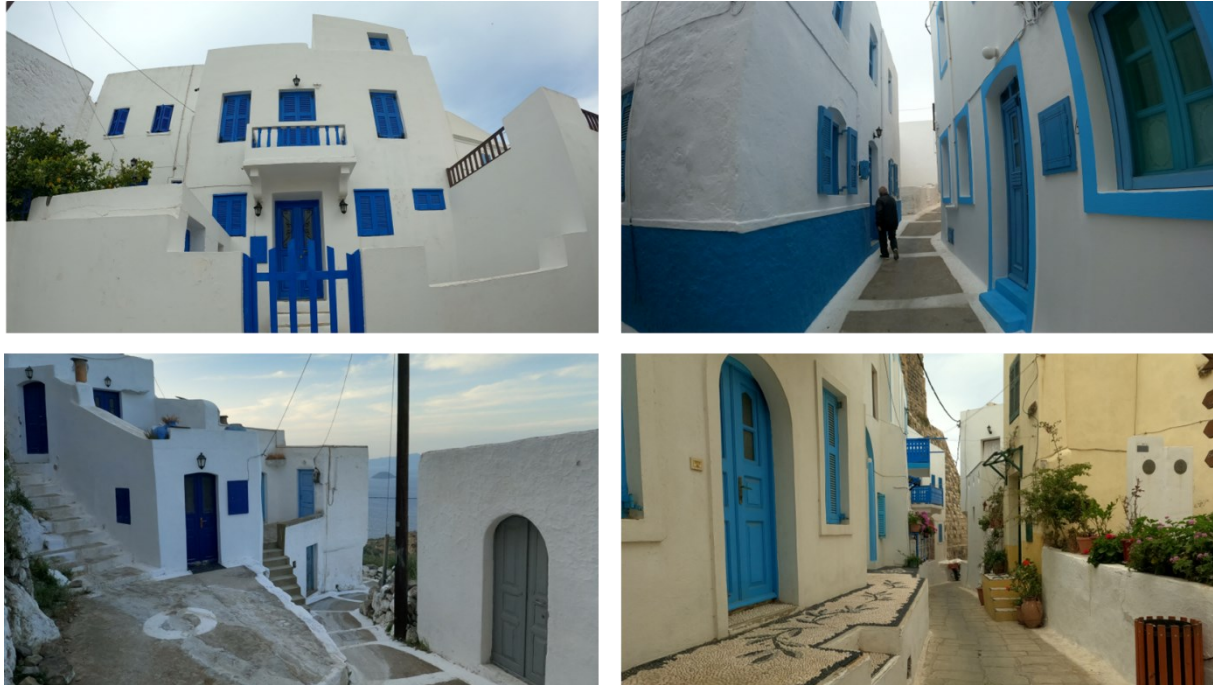
Fig. 2.4.6: Nisyrian settlements reflecting the typical characteristics of Dodecanese architecture.
